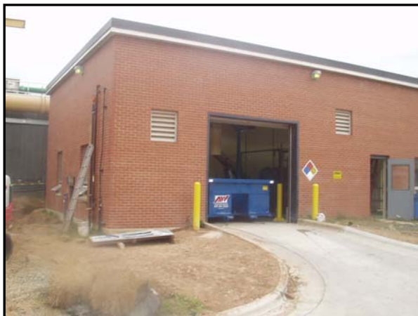
The dewatering system is housed within the old Dissolved Air Flotation Thickener Building at the Mason Farm WWTP.
