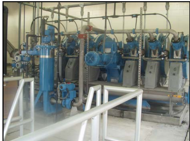
The new Fournier Rotary Press can meet our needs for a long time to come, as it has the capacity to meet our needs until the WWTP reaches a capacity of 18.5 MGD.
