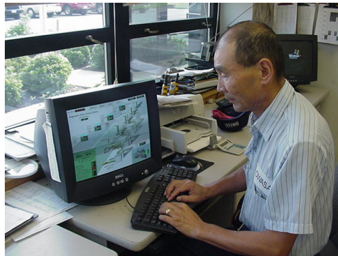
At our Mason Farm Wastewater Treatment Plant, we monitor operations with a computerized data acquisition and control system.
