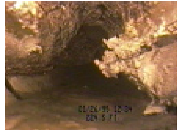
Above: Fat, oil and grease are beginning to accumulate in a sewer and restrict the flow of wastewater. This picture was taken with a special videocamera we use to inspect the sewer system.
