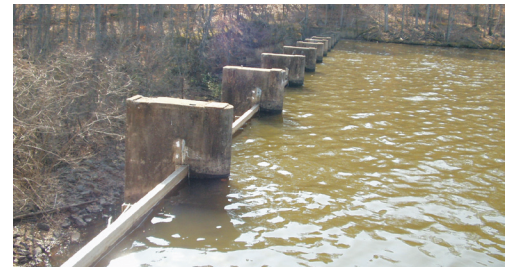
The dam at University Lake (early March)
