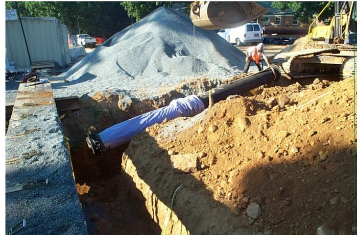
*In planning ahead for the reclaimed water system, the University has already begun to install reclaimed water pipes as part of construction on the main campus.*
