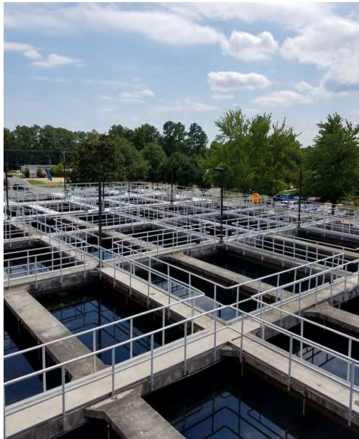
Water Treatment Plant Sedimentation Basins
