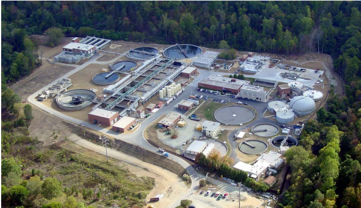
The Mason Farm Wastewater Treatment Plant following a three-year, $50 million upgrade and expansion project substantially completed in July, 2007
