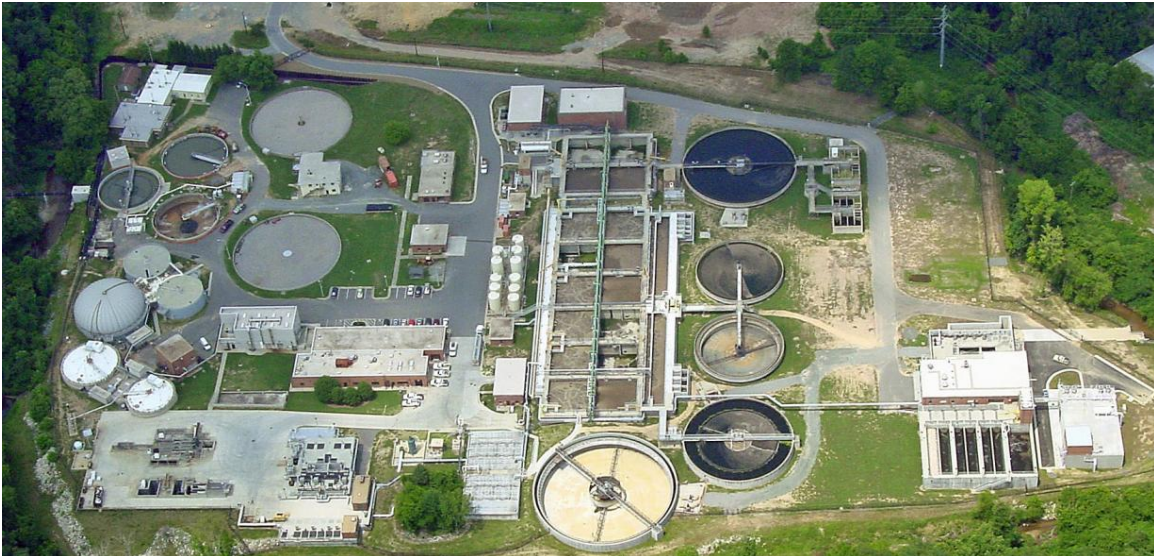
Mason Farm Wastewater Treatment Plant
