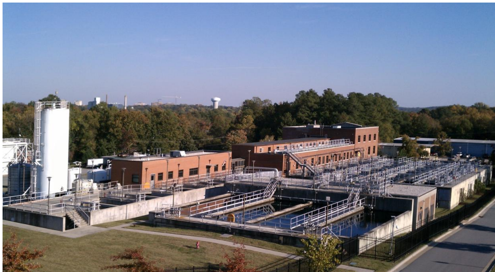
Jones Ferry Road Water Treatment Plant
