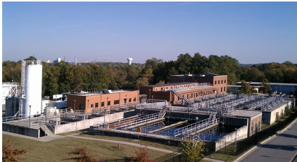
Jones Ferry Road Water Treatment Plant
