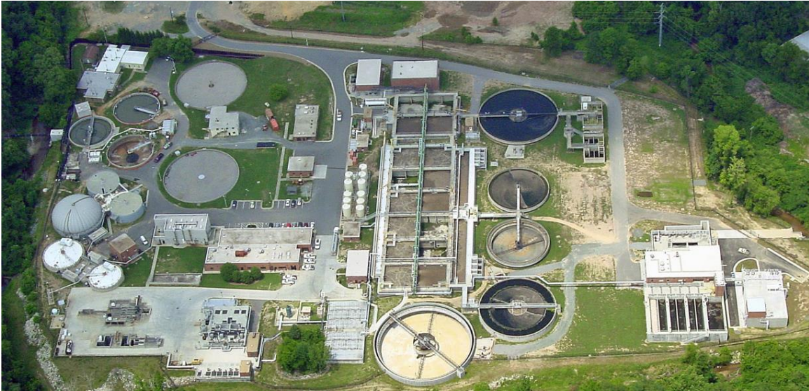
Mason Farm Wastewater Treatment Plant
