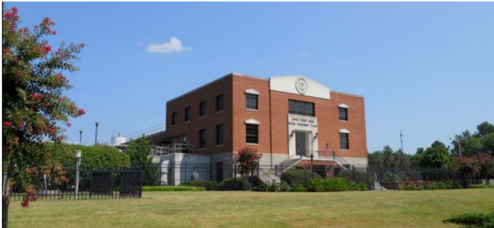
Jones Ferry Road Water Treatment Plant
