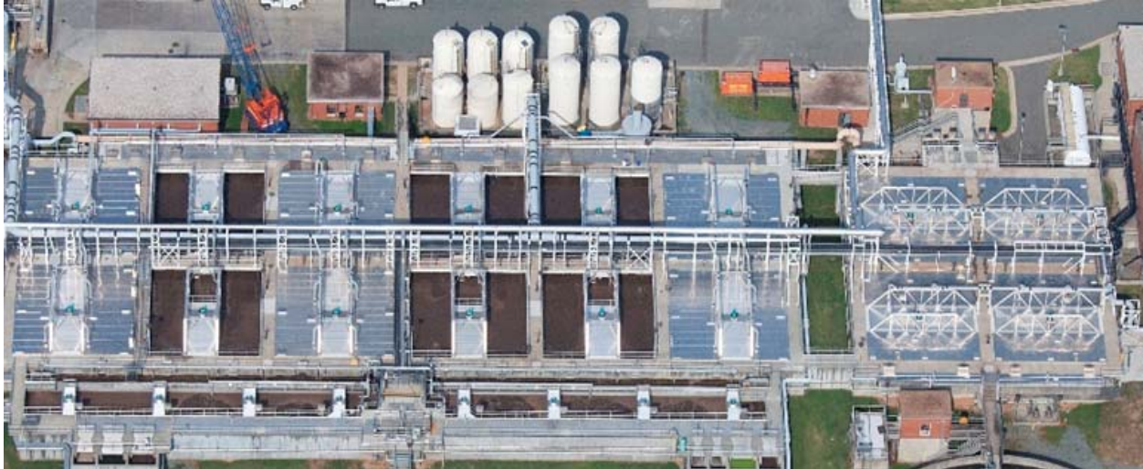
Aerial photo of the aeration basins at OWASA's Mason Farm Wastewater Treatment Plant
