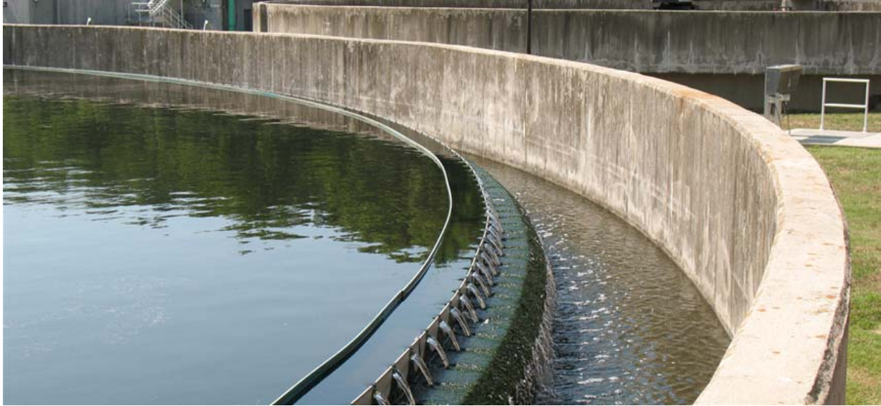
Mason Farm Wastewater Treatment Plant
