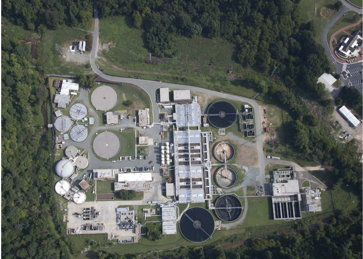
Mason Farm Wastewater Treatment Plant
