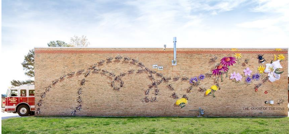
Carrboro Fire Station
