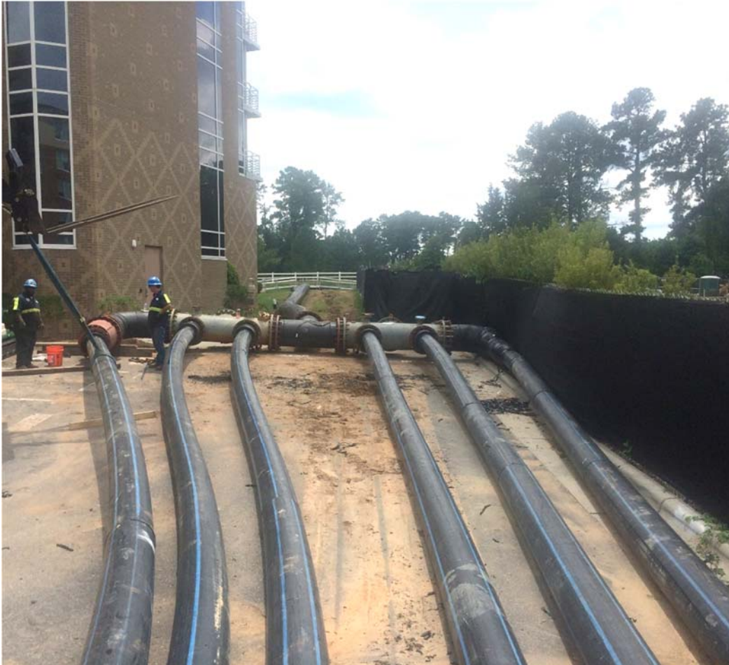
Bypass Piping During Construction on OWASA's Most Critical Pump Station
