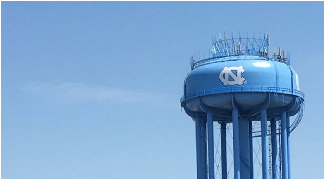
Elevated Water Storage Tank on the UNC Campus
