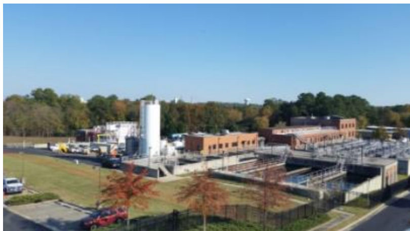
Jones Ferry Road Water Treatment Plant
