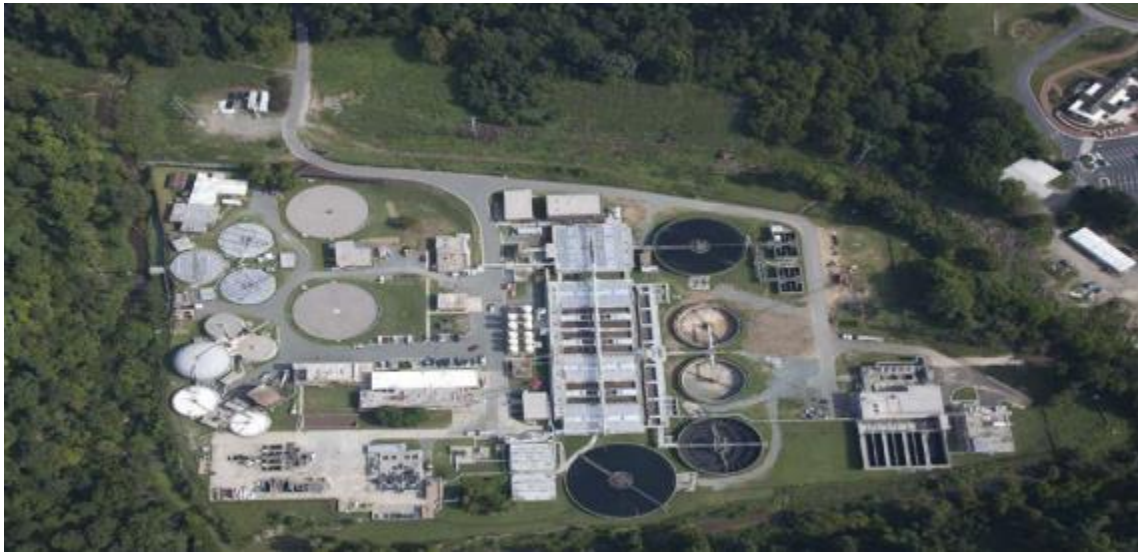
Mason Farm Wastewater Treatment Plant
