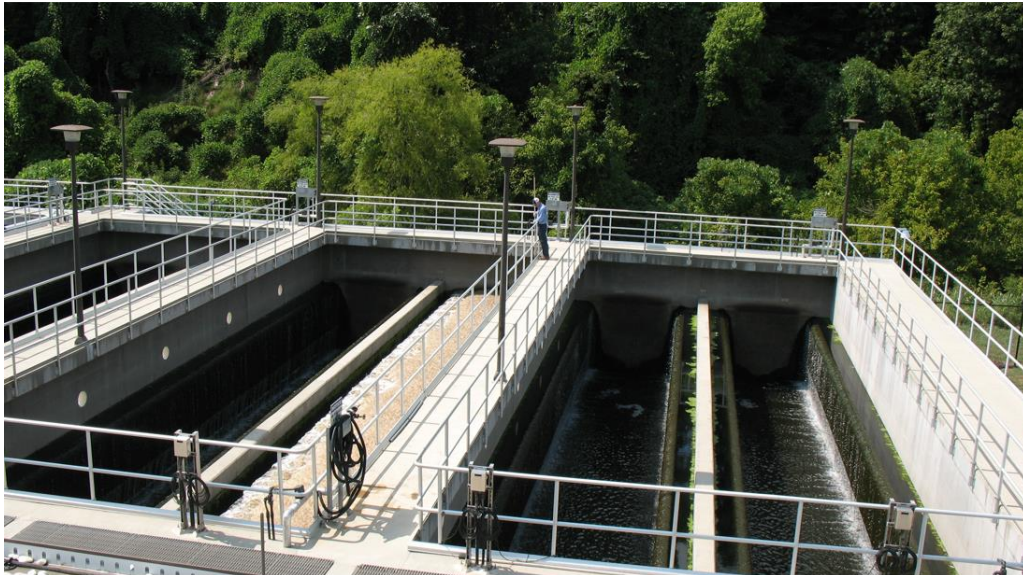
Mason Farm Wastewater Treatment Plant
