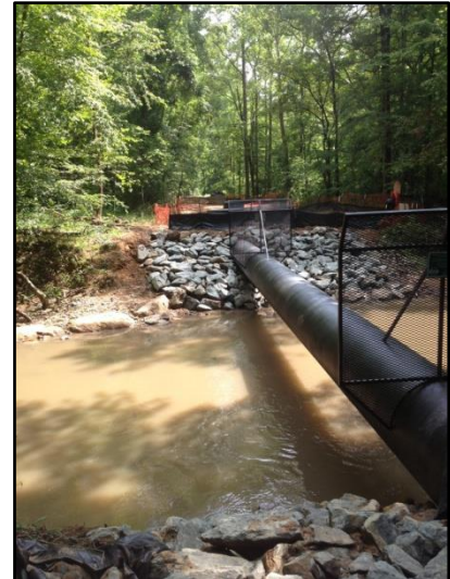
Morgan Creek Aerial Crossing with Pedestrian Barricades
