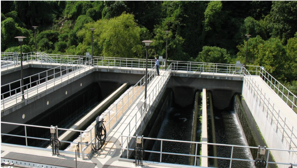
Mason Farm Wastewater Treatment Plant
