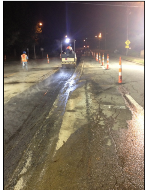
Paving over the water main installation at night in South Estes Drive
